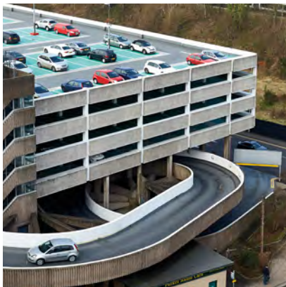
Above: One of the town centre's car parks.
