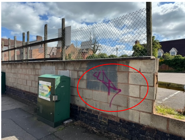
RAILWAY ROAD, NEAR JUNCTION OF REDDICROFT
